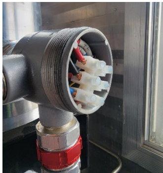
Conductor Cable Termination in Junction Box
